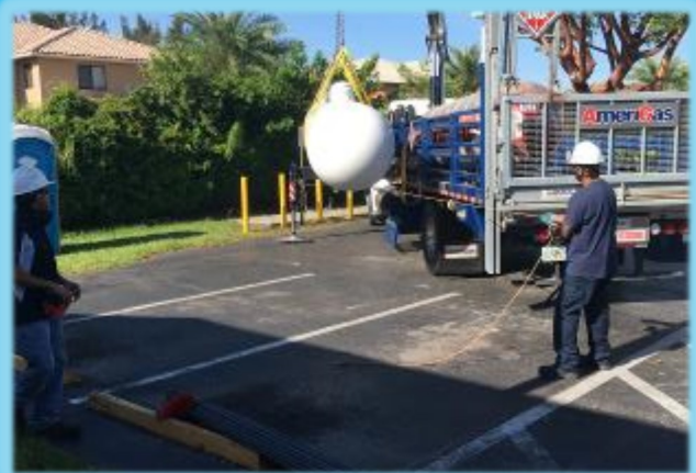
Pictured above: Removal of the now obsolete propane tanks.
