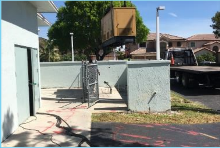
Pictured above: Removal of the existing generators.
